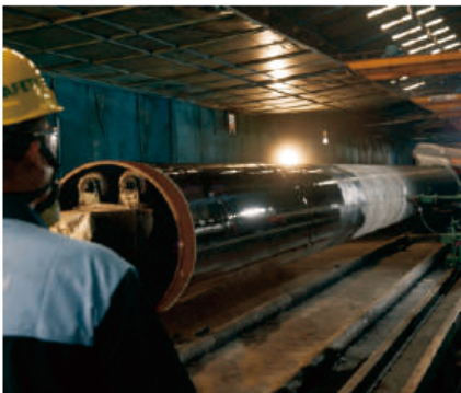
External Epoxy Coating
