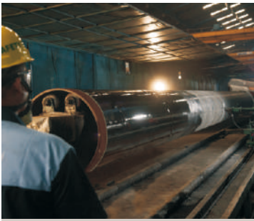
External Epoxy Coating
